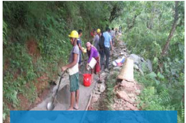
Irrigation canal progressing
